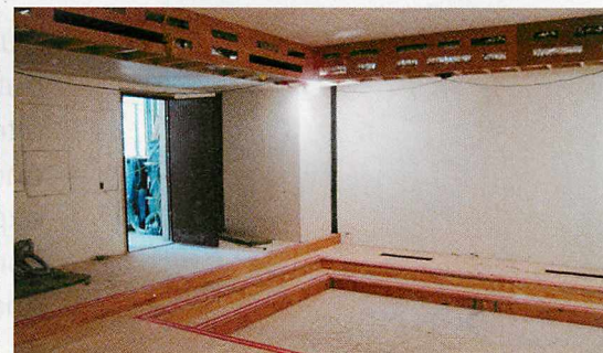
• Left: Phase one of a "lounge-cinema" designed by PMI, Ltd., showing the framing with isolated double-wall construction and spring-suspended ceiling structure. The internal walls do not connect with the ceiling but are instead tied back to the external load-bearing wall with rubber isolators. Right: Phase two shows the room after the drywall has gone up. The finished room is pictured at the top of the page.
