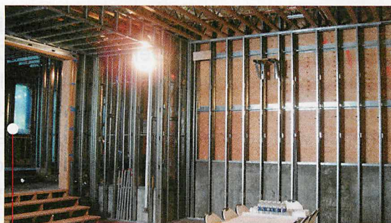
• Left: Phase one of a "lounge-cinema" designed by PMI, Ltd., showing the framing with isolated double-wall construction and spring-suspended ceiling structure. The internal walls do not connect with the ceiling but are instead tied back to the external load-bearing wall with rubber isolators. Right: Phase two shows the room after the drywall has gone up. The finished room is pictured at the top of the page.
