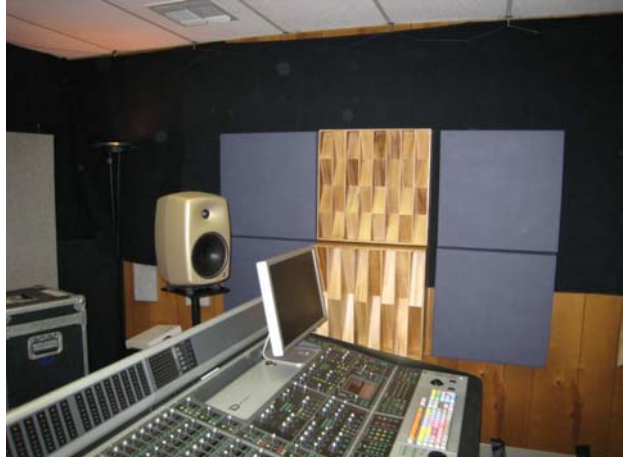
The right wall featured a blend of StudioPanel Pro absorbers and diffusers from MSR.
