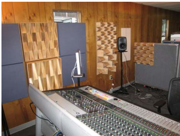
The back portion of the 53 foot long trailer was divided from the mix area by IsoPanels, visible here above and to the left of the mixing chair.
